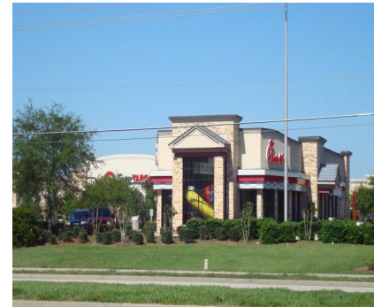
A well maintained commercial property.
