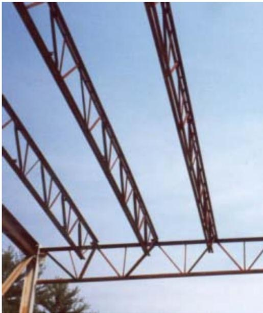
Bar Joist . **This type does not apply to the above rule.**
