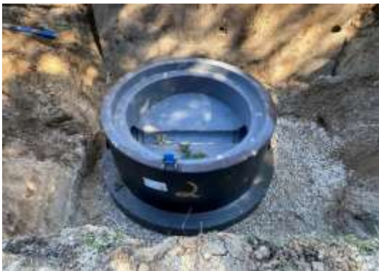
Photo of new manhole set on Ponce De Leon Circle as part of the septic to sewer project
