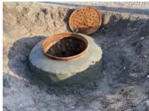
Photo of new manhole set on Ponce De Leon Circle as part of the septic to sewer project
