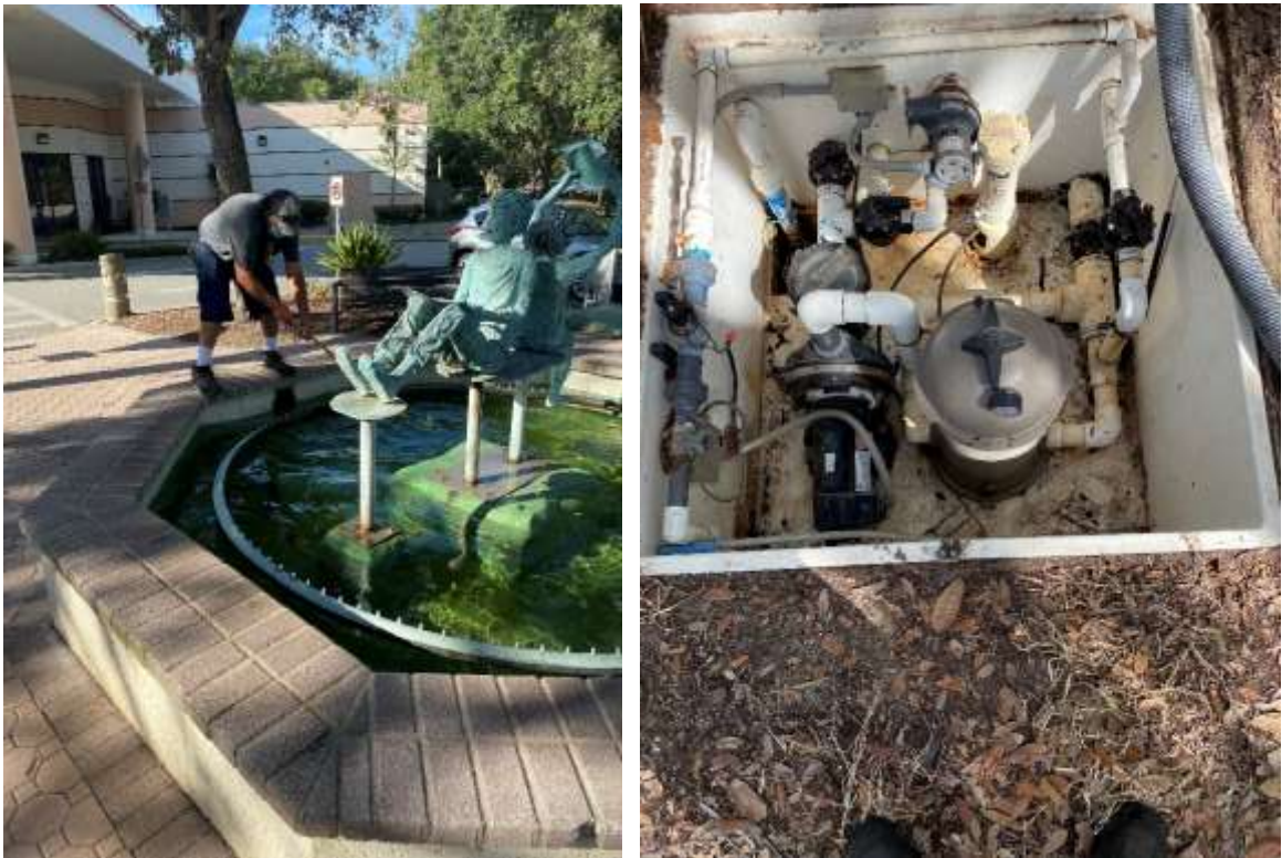
Photos of staff cleaning the library fountain and pump house
