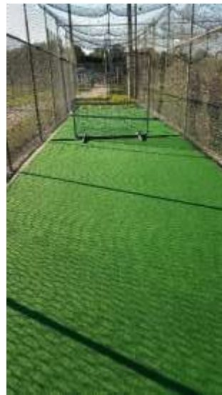
Photo of new turf after installation
