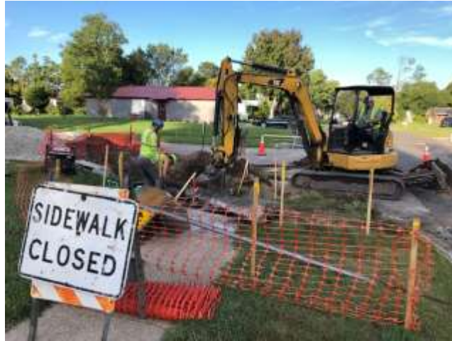
Photo of storm pipe being installed on Pagano Court
