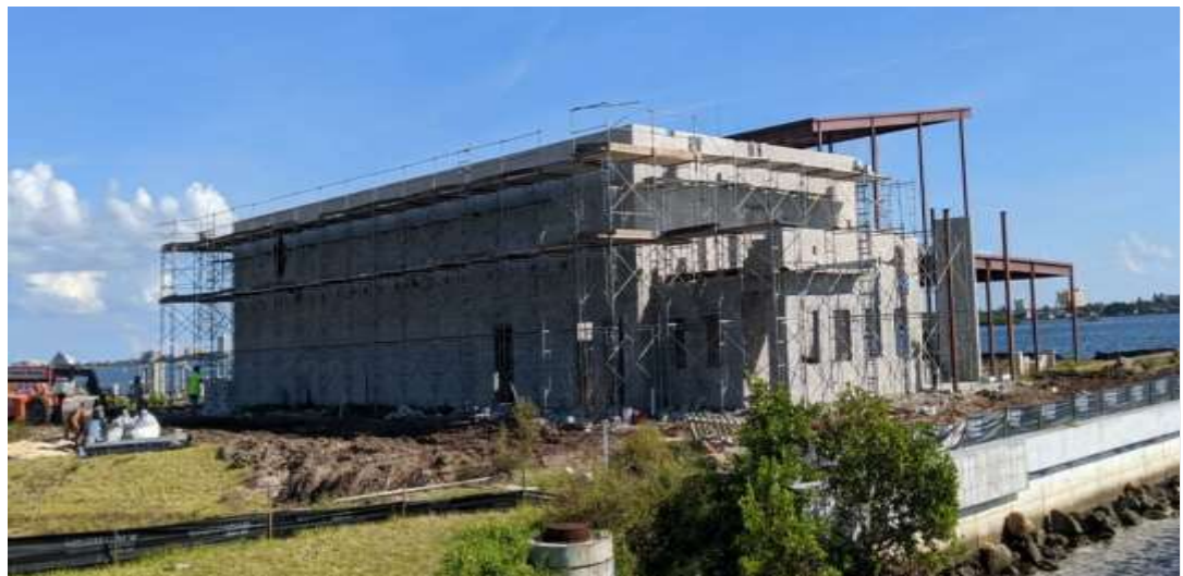
Photo of Fysh Bar & Grill Restaurant under construction
