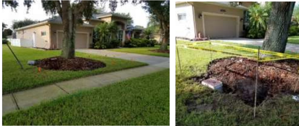
Photos of repaired reclaim water service in Sabal Creek
