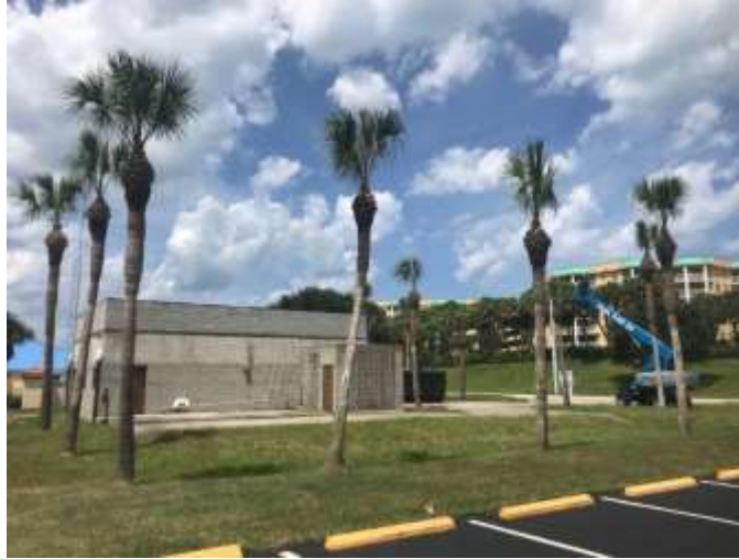
Photo of the Palms that were trimmed at the Ponce Inlet Lift Station
