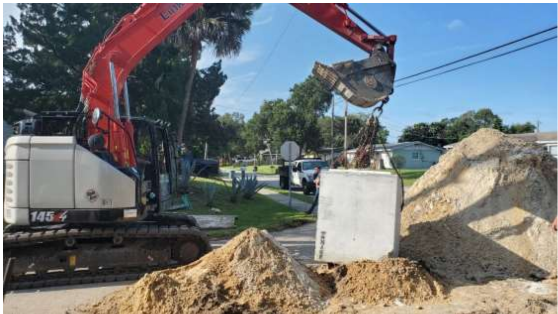
Photo of stormwater inlet being set by the contractor
