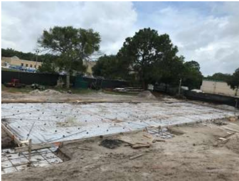
Photo of the storage building foundation
