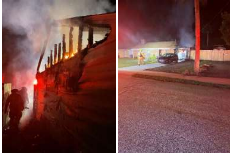
Photos from Lafayette Street structure fire
