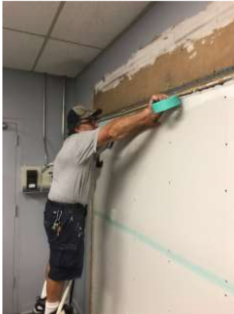
Photo of the staff repairing drywall at Public Works
