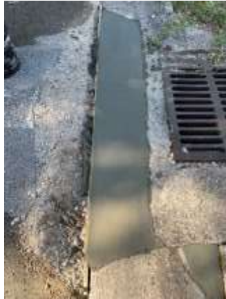
Photo of repaired curbing at 28 Golden Gate Circle
