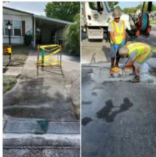
Photo of Field Ops crew cutting the driveway on Greenfield Dr.
