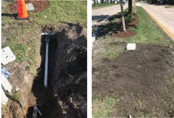
Before and after photos of the irrigation repairs on Ridgewood Ave.
