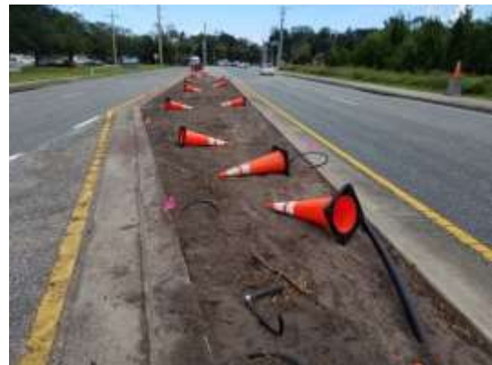
Photo of irrigation installed in median near Spruce Creek Road
