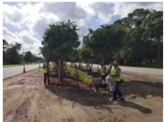
Photo of work crew placing mulch in median
