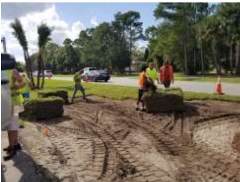
Photo of sod being installed on Dunlawton Ave. median
