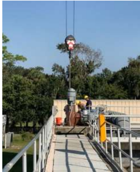
Photos of a rebuilt internal recycle pump being installed at the WRF.
