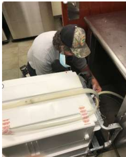
Photo of Staff Installing a New Dishwasher at Fire Station 75
