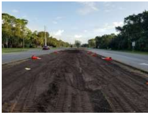
Photo of median east of Jackson Street stripped of vegetation
