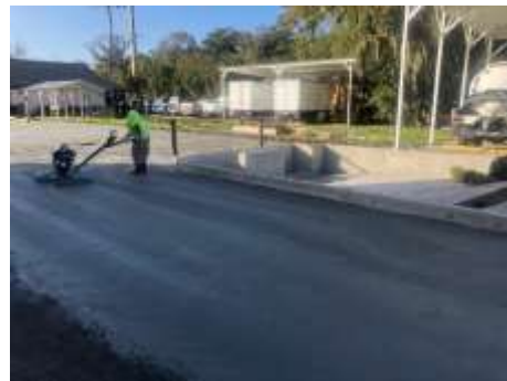
Photos of the Sludge Trailer Storage Lot project concrete being finished by the contractor.
