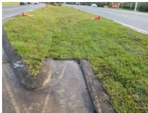
Photo of sod installation in first median east of Nova Road
