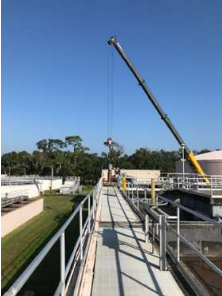
Photos of a rebuilt internal recycle pump being installed at the WRF.
