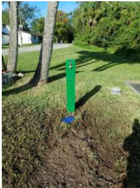
Photo of new water sampling station at Taylor Rd. and Country Lane
