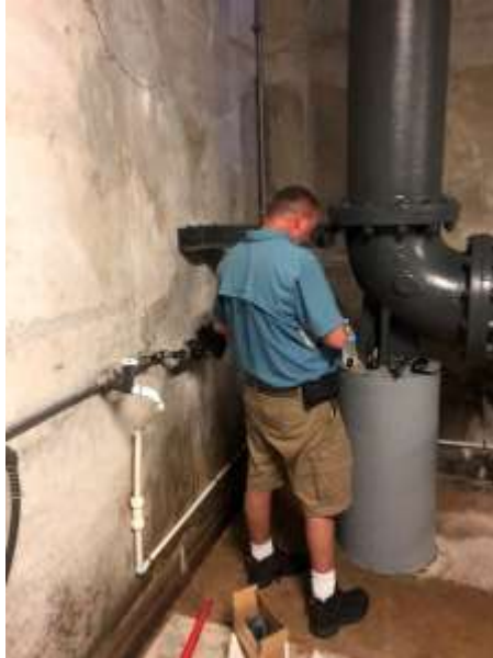
Photo of repairs to a backflow device at Ponce Lift Station
