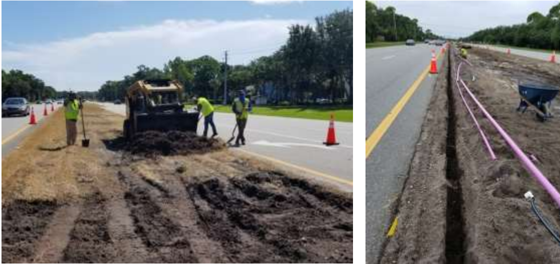
Photos of work being done to the Dunlawton Ave. medians.
