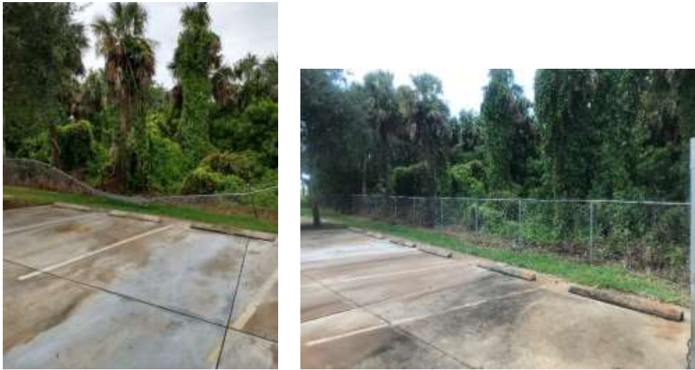
Photo of before and after fence replacement
