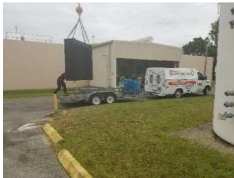
Photos of generator being repaired at the WRF
