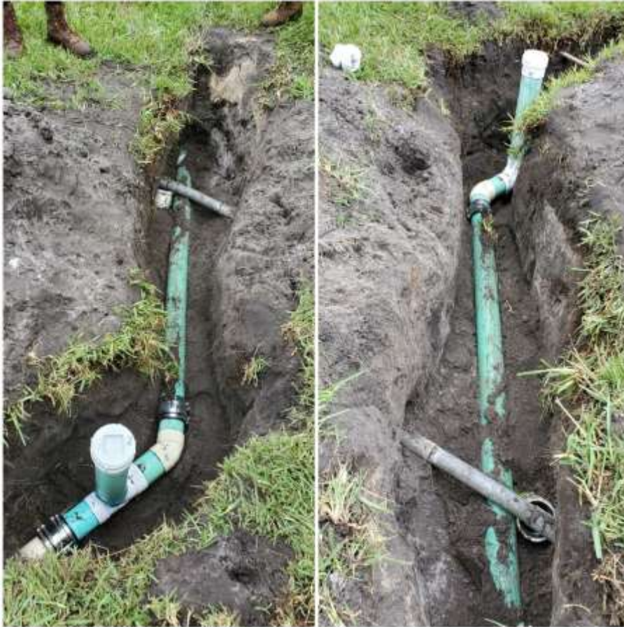
Photo of repaired sewer lateral on Chickadee Dr.
