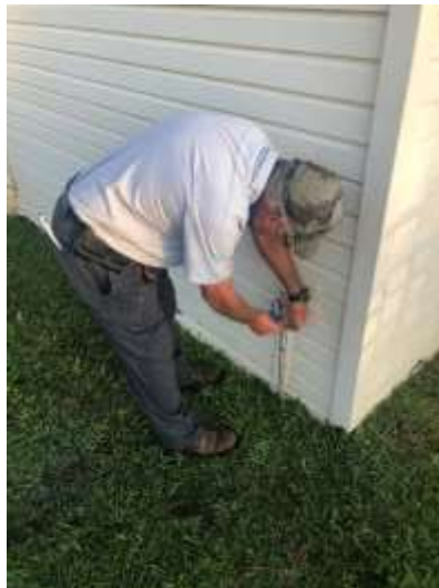
Photo of repairing faucet
