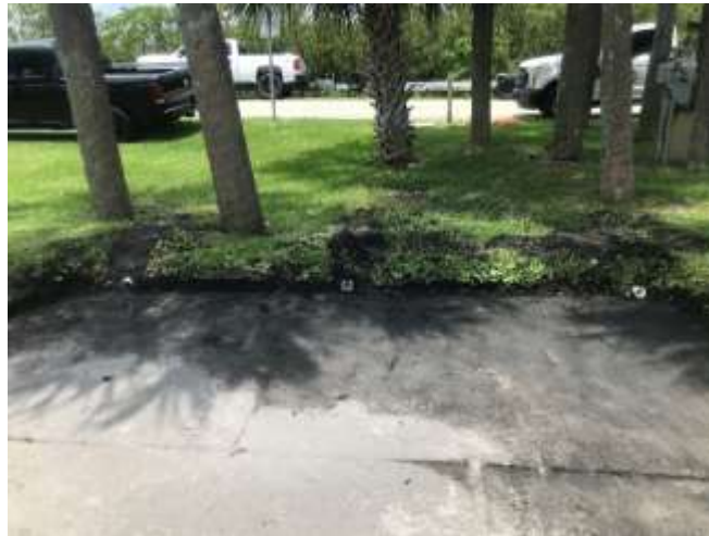
Photo of after drainage was installed
