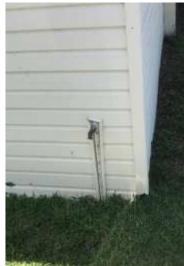
Photo of repaired faucet
