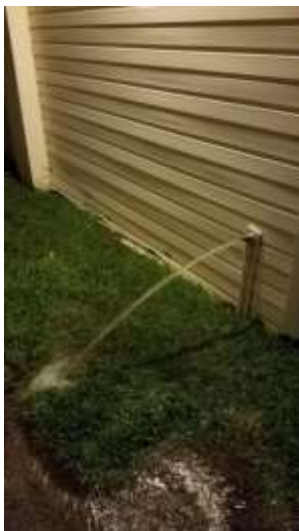
Photo of broken faucet
