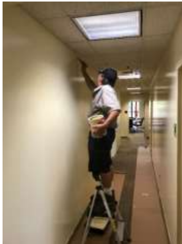
Photo of Staff Painting Hallway Walls at City Hall
