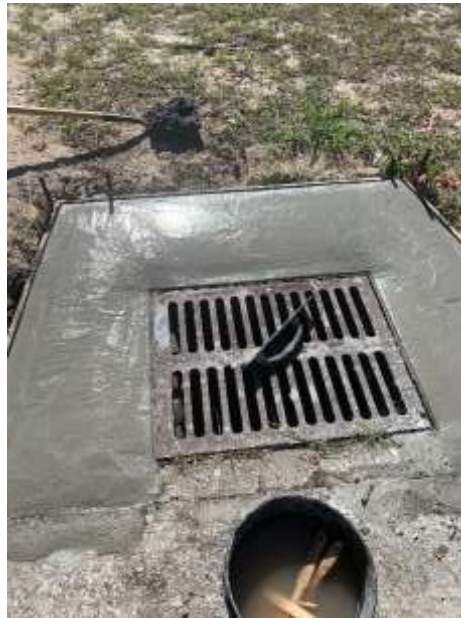
Photo of Concrete Basin at 1134 Viking Drive
