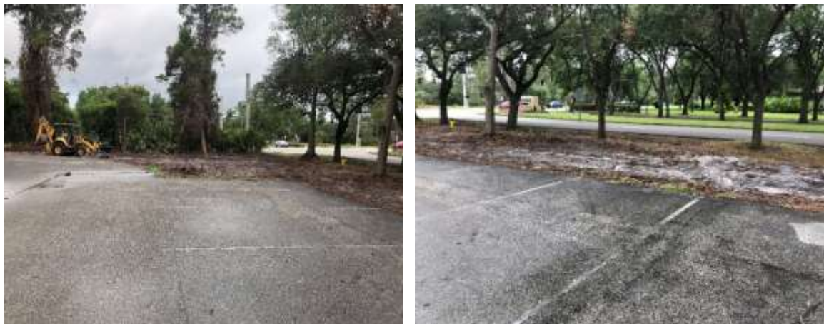
Photos of Fire Station 73 Parking Lot being prepped for Hydroseed
