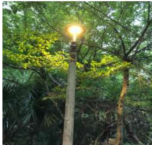
Photo of light pole repairs completed
