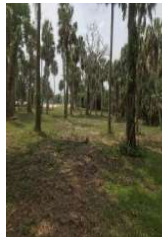
Photo of completed mowing
