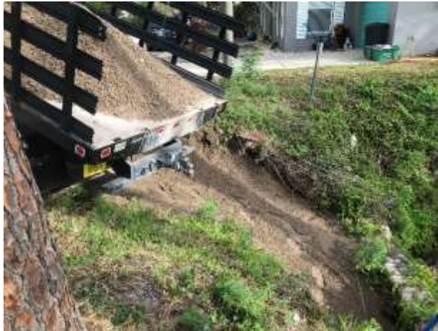
Photo of Staff filling in the washed-out spillway on Alexander Ave
