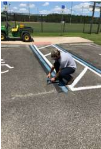
Photos of crew repainting the handicap lines in the parking lot. Photo of repainting completed
