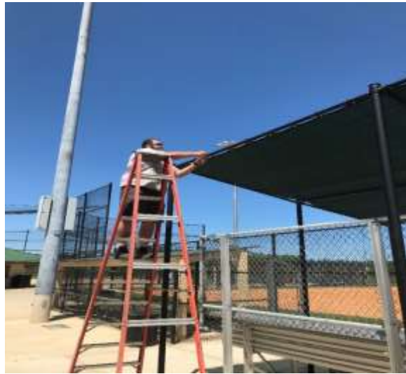
Photo of new sunshades being installed
