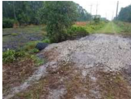
Photo of repaired drainage culvert off Shunz Rd.
