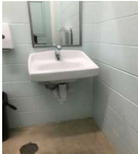
Photo of new sink installed
