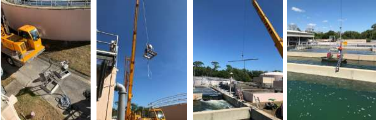
Photo of new chlorine mixers being installed at the WRF
