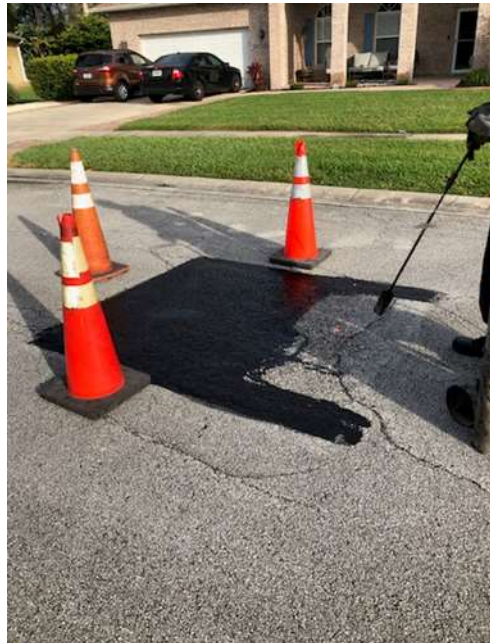
Photo of the asphalt repair in the Sterling Chase Subdivision
