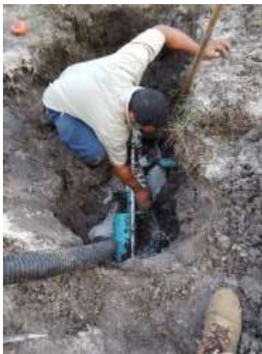
Field Ops crews repaired a broken irrigation line on at Cypress Head Golf Course
