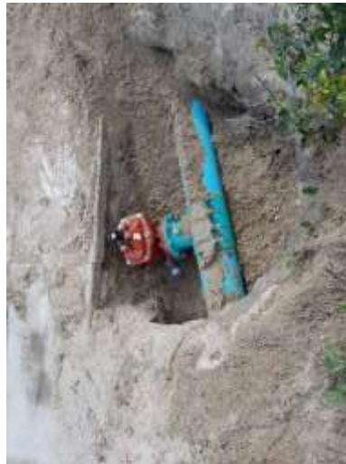
Field Ops crews performed a 6” tap in Daytona Beach Shores for a new development
