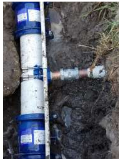
Field Ops crews repaired a broken irrigation line on at Cypress Head Golf Course
