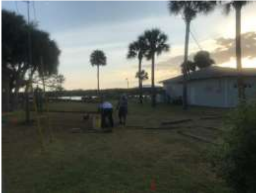
Photo of crew working on Split Rail Fence
