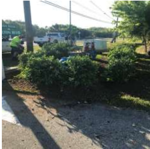
Photo of the new plants around the Master Meter at Lamplighter
