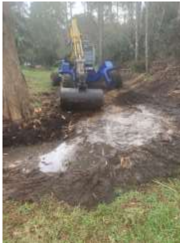
Photo of the Kaiser working on Pelham Drive Ditch
