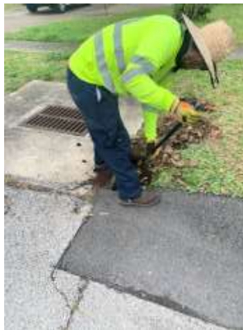
Photo of employee, Anthony, repairing a failed storm drain
