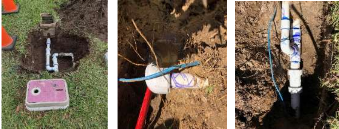
Photos of irrigation pipe repairs
