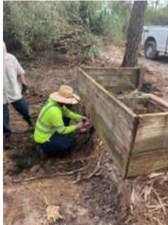
Photo of Anthony repairing the skimmer boards
