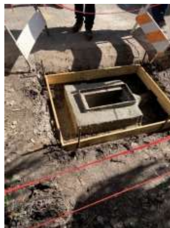
Before, during, and after repairs of a failing catch basin
