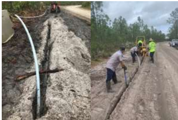
Photos of crew laying pipe
