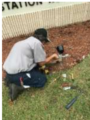
Photo of employee repairing sign lights
