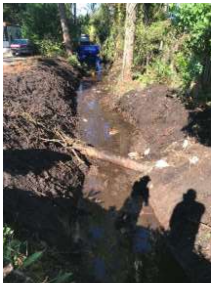
Photo of the Kaiser clearing out the Tanglewood ditch
