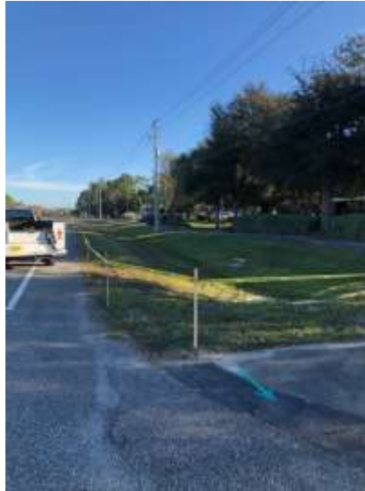
Photo of staked off right of way along Dunlawton Ave.
