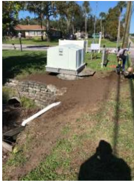
Photos of installed pipe
