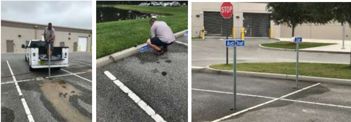
Photos of newly installed signs
