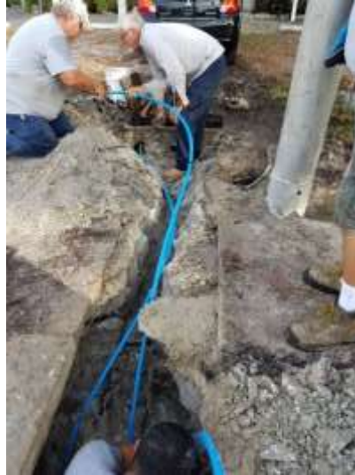
Photo of Field Ops staff replacing service lines on Charles Street
