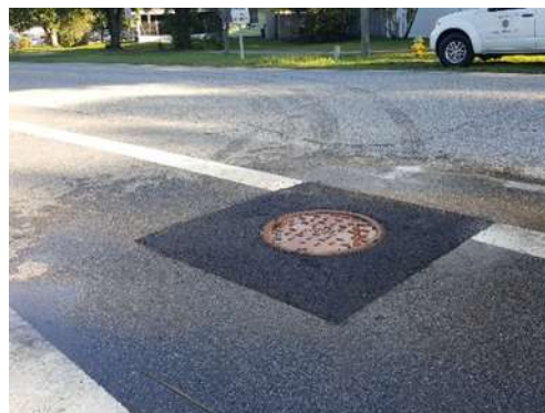
Photo of demonstration of a paving patch material for Field Ops
