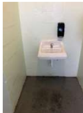
Photo of the new replacement sink
