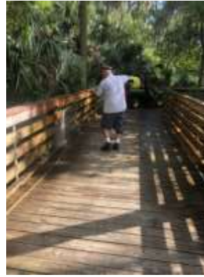
Picture of the deck being pressure washed
