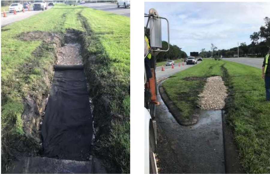
Photos of swale rehab in a Dunlawton Avenue median
