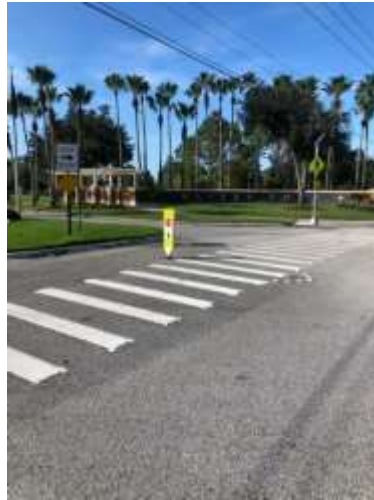
Photos of signs installed on Waters Edge Boulevard
