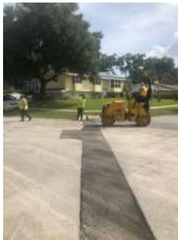
Before and after photos of asphalt patch
