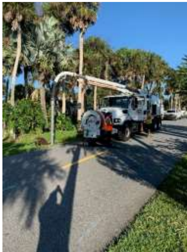
Photo of vaccon cleaning catch basin on Riverside Drive
