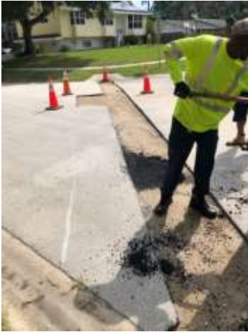
Before and after photos of asphalt patch
