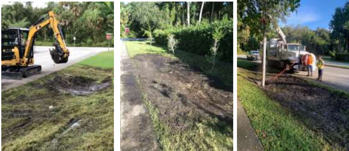
Photos of regraded swale on Woodbriar Trail and North Swallowtail Drive
