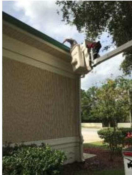
Photo of employee checking rain gutters
