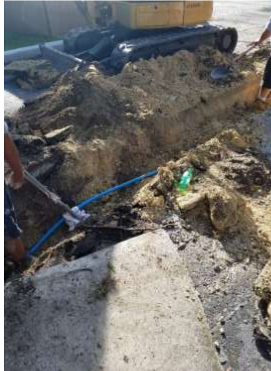
Photo of new service line that distribution crews installed in Trailwood
