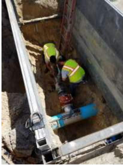
City staff performing a waterline tap in King's Landing.
