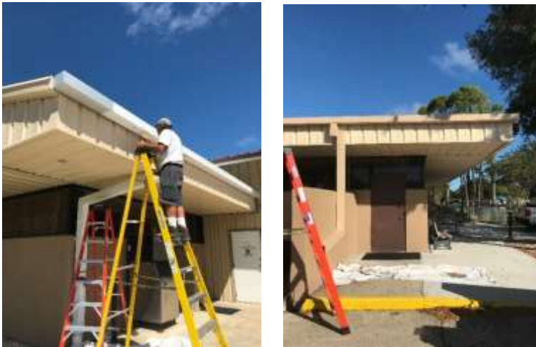
Photos of employee painting Public Works gutters
