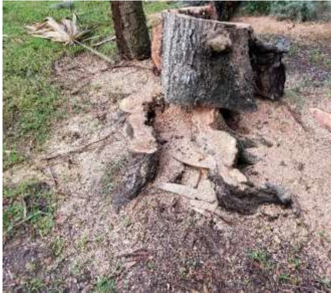
Photo of the large tree being removed
