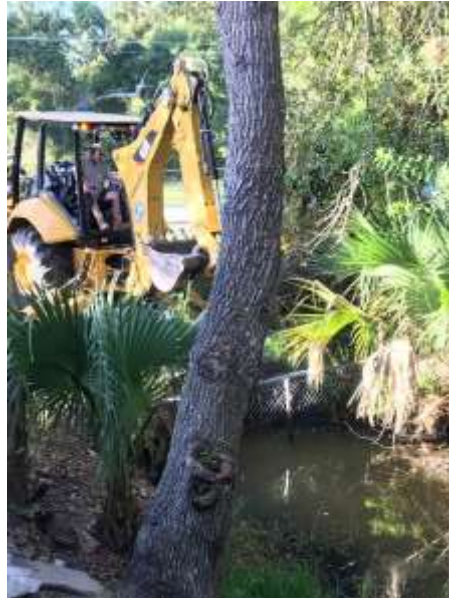
Photo of the ditch being cleaned out
