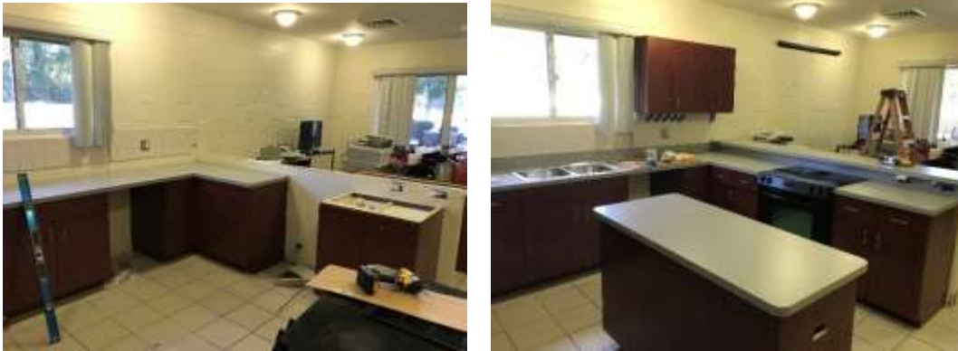
Photos of Fire Station 74 remodel
