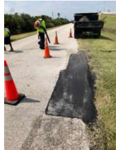
Before and after photos of shoulder repair by Deck Down Under
