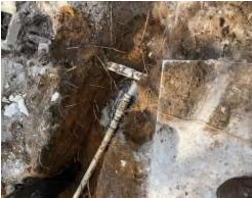
Photo of broken sprinkler under sidewalk Photo of repair completed at Seemore Dog Park
