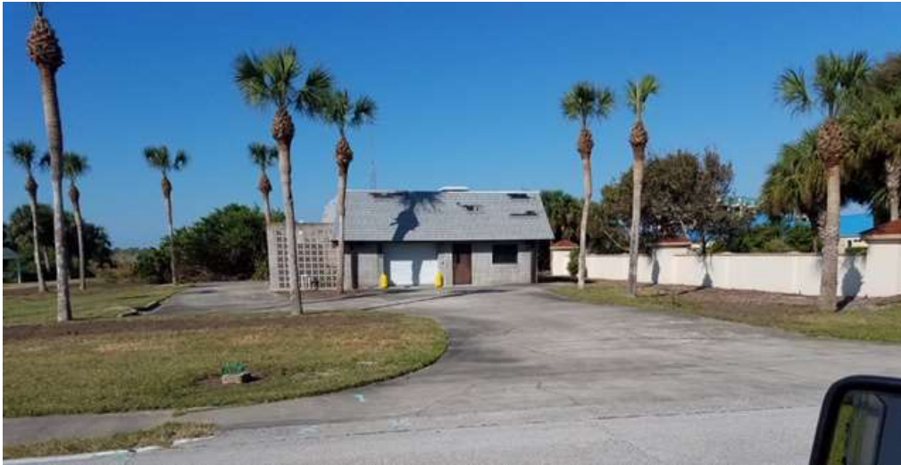
Photo of Ponce Inlet master lift station after Public Works trimmed the palm trees
