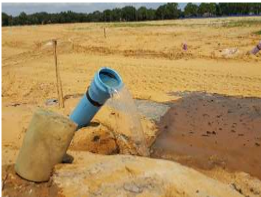
Photo of water and reclaimed mains being flushed “pigged” in Kings Landing
