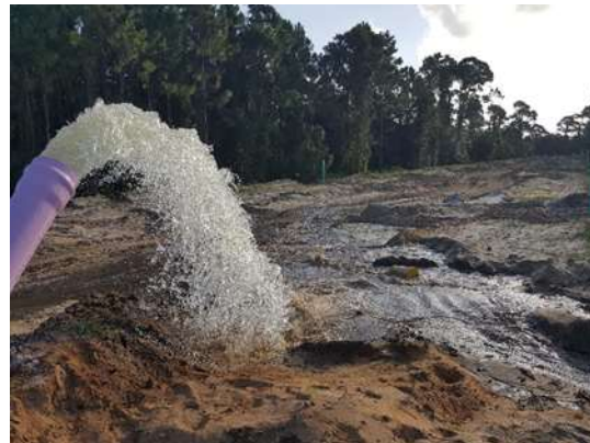
Photo of water and reclaimed mains being flushed “pigged” in Kings Landing
