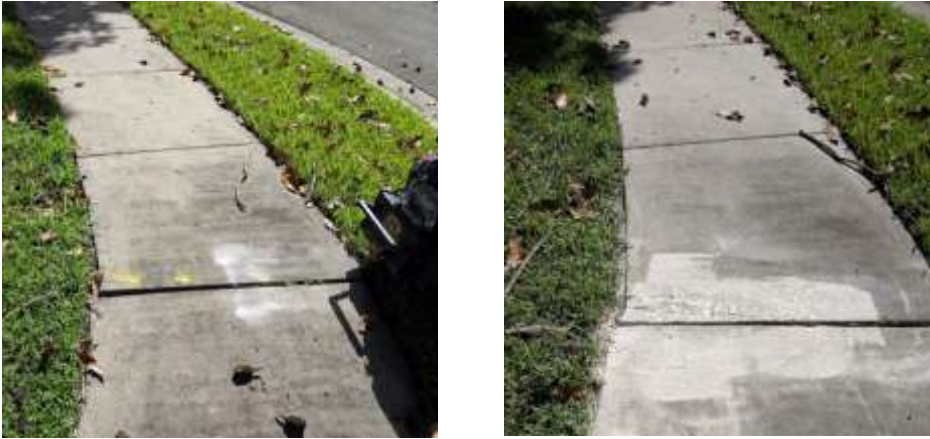
Before and after photos of sidewalk grindings
