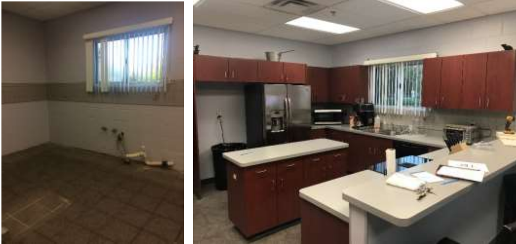
Before and after photos of Fire Station 74 Kitchen
