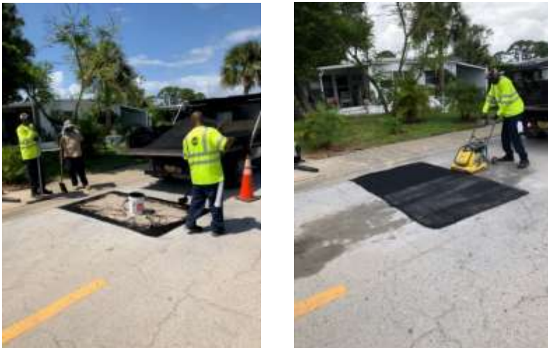
Before and After photos of asphalt repairs
