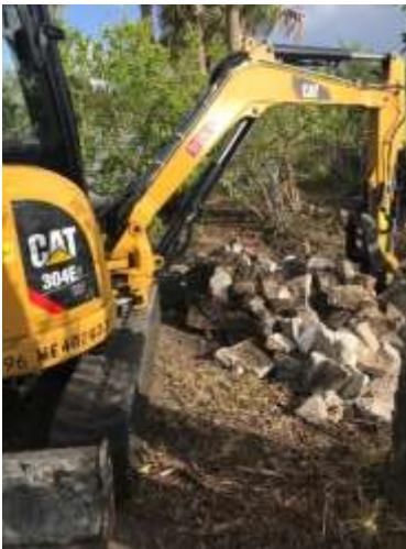
Photo of the mini excavator stabilizing the bank
