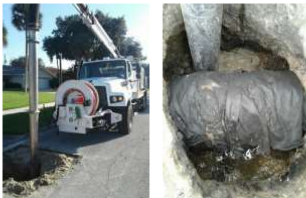
Photo of Vac-con truck and stormwater pipe
