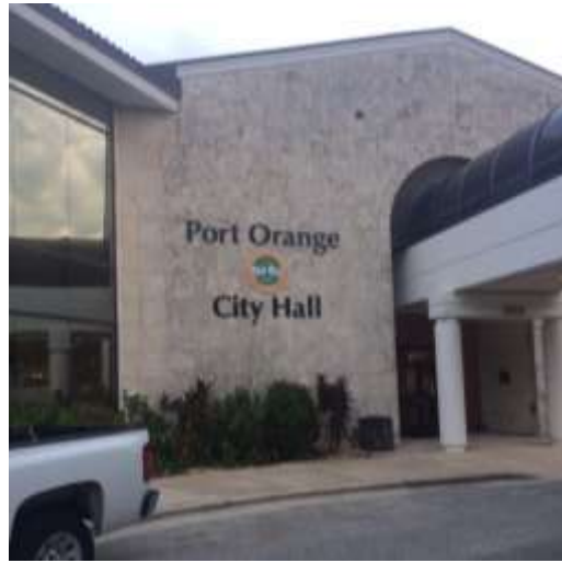
Port Orange City Hall Sign installed on the building
