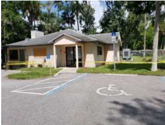
Photo of newly installed sod at the Central Lab building
