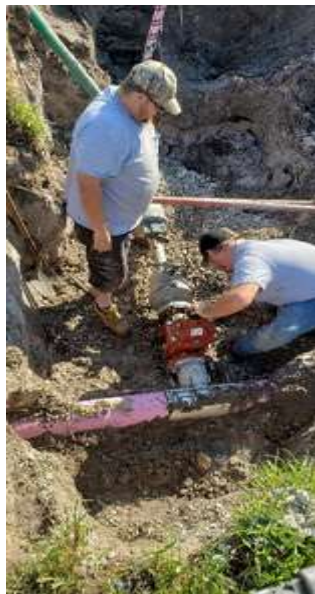
Photo of staff performing a reclaimed tap at Crane Lakes and replacing a 2" PVC reclaimed line at the YMCA
