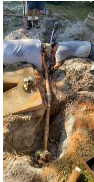
Photo of staff performing a reclaimed tap at Crane Lakes and replacing a 2" PVC reclaimed line at the YMCA
