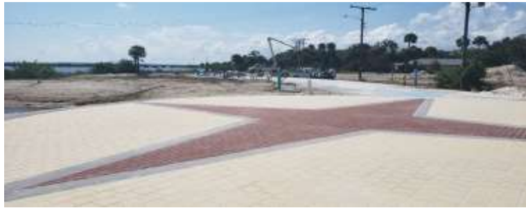
Photo of public trail with decorative pavers installed
