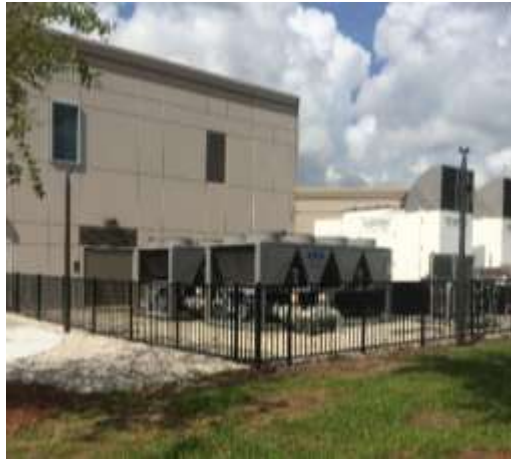
Photo of newly installed fence at Police Department
