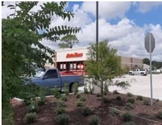
Photo of AutoZone (front and side of building) and parking lot.
