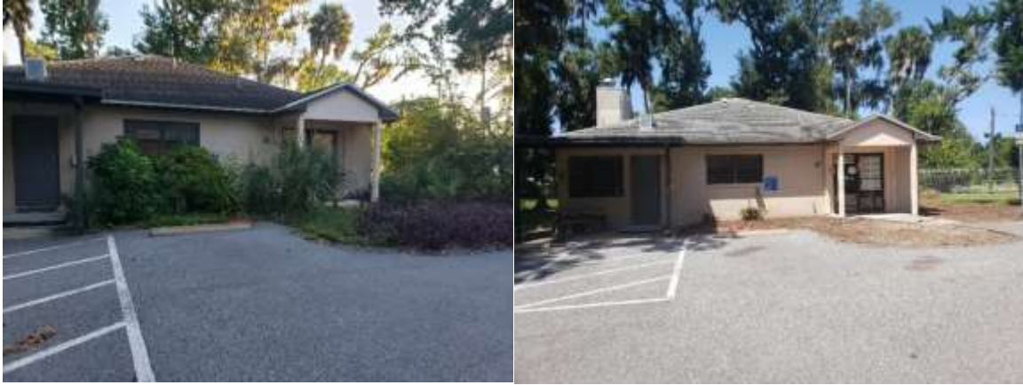
Photo of the laboratory exterior before and after clean-up
