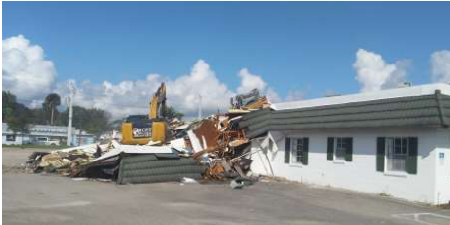
Photo of demolition of the Cardwell Funeral Home
