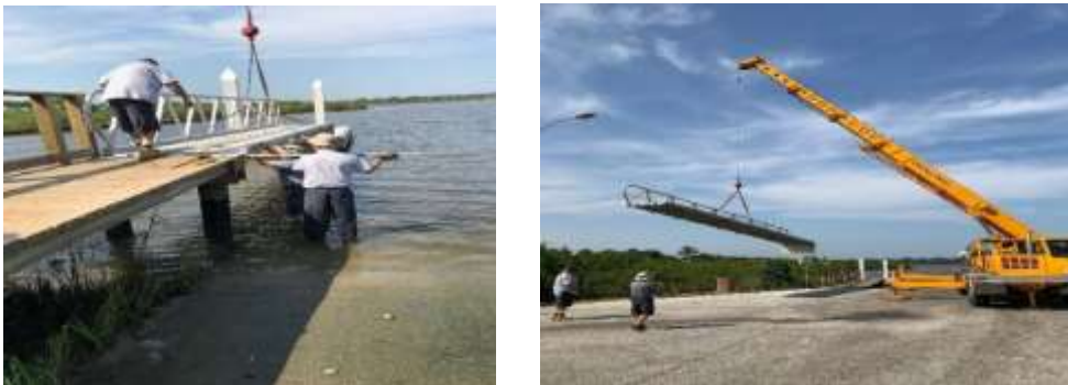
Photos of crew removing and replacing Gangways at Causeway Park
