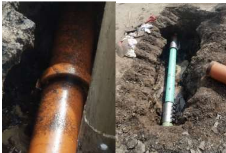
Photo of clay sewer line repair performed on Farmbrook Rd.
