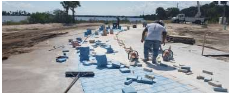
Photo of public trail with decorative pavers being installed
