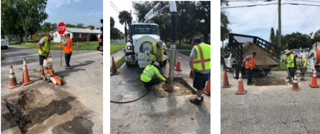
Photos of the Drainage crew repairing a pipe on Charles Street
