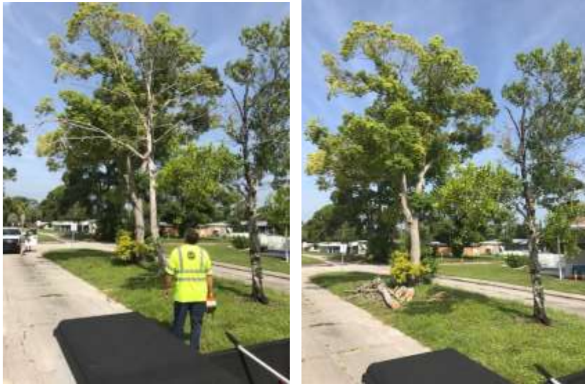
Before and After photos of tree removal
