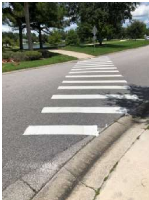
Photo of newly painted crosswalk
