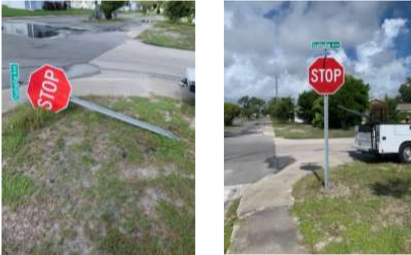
Before and After photos of a repaired sign
