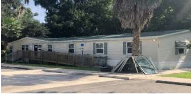
Photo of Historical Trust Building with new windows
