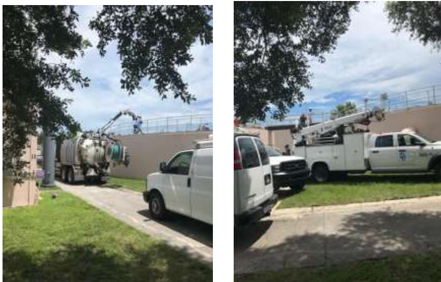
Photo of cleaning the North clarifier at the WRF
