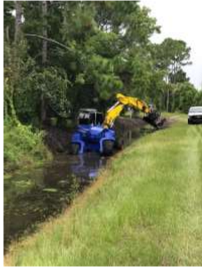
Photo of the Kaiser working in the Cross Creek ditch
