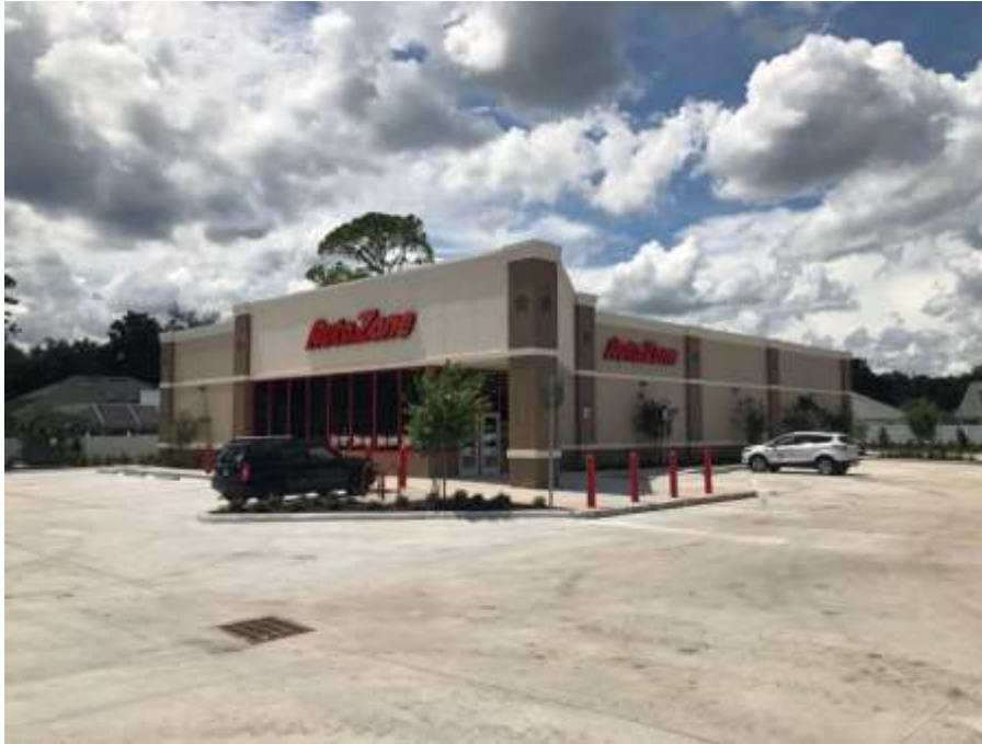
Photo of AutoZone (front and side of building) and parking lot
