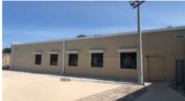
Photo of the paint job at the YMCA
