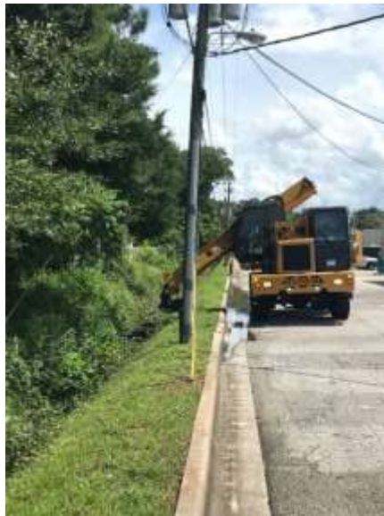
Photo of the Grad-All working in the Publix ditch
