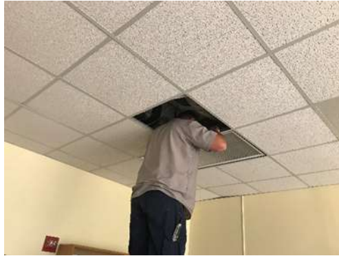
Photo of employee inspecting the ceiling
