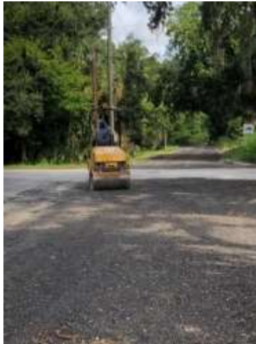
Photo of employee rolling Westridge Avenue
