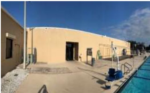
Photo of the YMCA pool area
