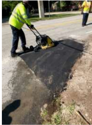
Before and After photos of employees completing a utility patch
