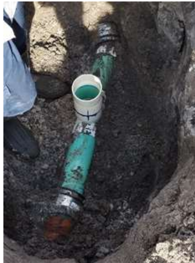
New Sewer Cleanout Installed to a Home on Isabelle Avenue
