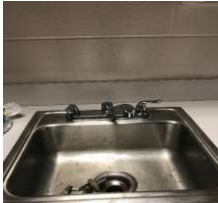
Photo of newly installed faucet
