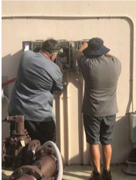
Photo of John Baller and Rob Kuhn installing new safety switches at the WRF
