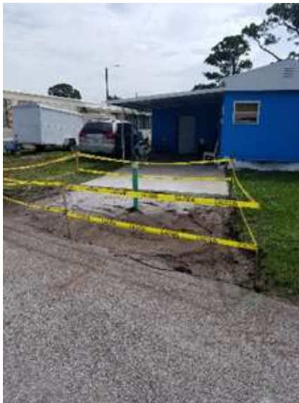
New Sewer Cleanout Installed to a Home on Isabelle Avenue
