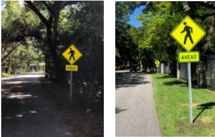
Photos of pedestrian signs installation on old Sugar Mill Road
