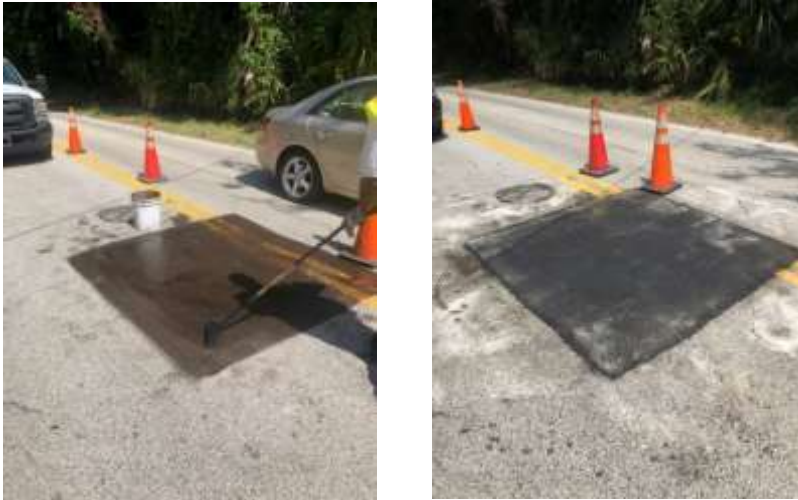
Photos of Herbert St. asphalt repairs
