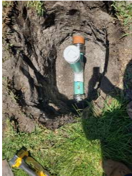
Photos of sewer clean out installed on a clay sewer line
