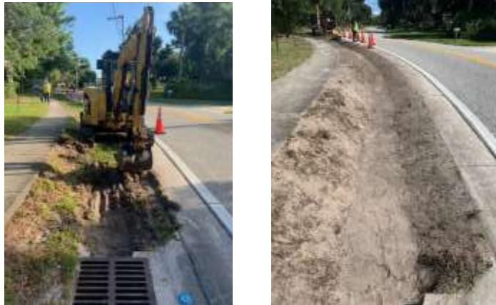
Photos of pipe install on Boggs Ford Rd
