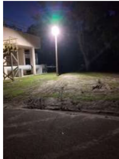
Photo of new light fixture installed
