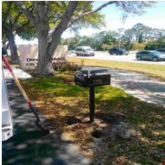
Photo of New Mailbox installed at DLH City Center Annex
