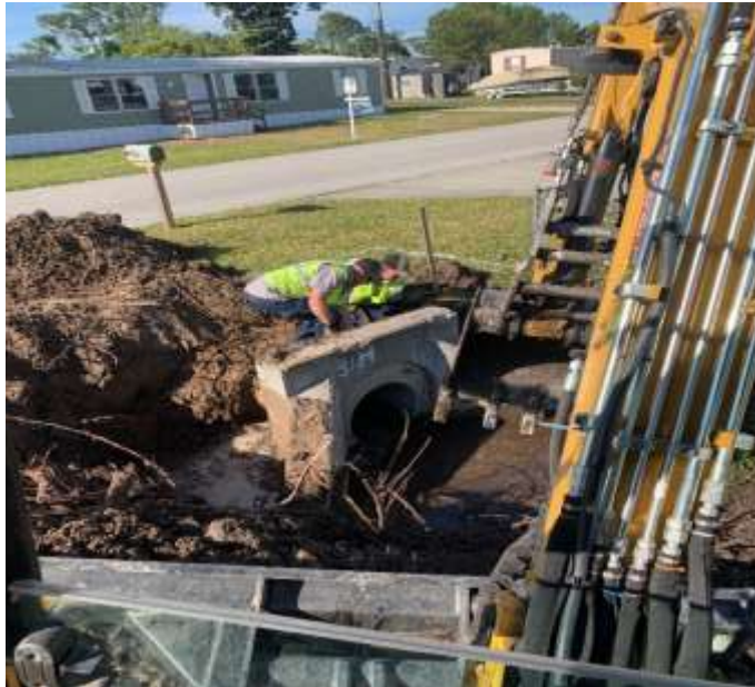
Photo of Staff working on the Turton and Barhydt Drainage Project
