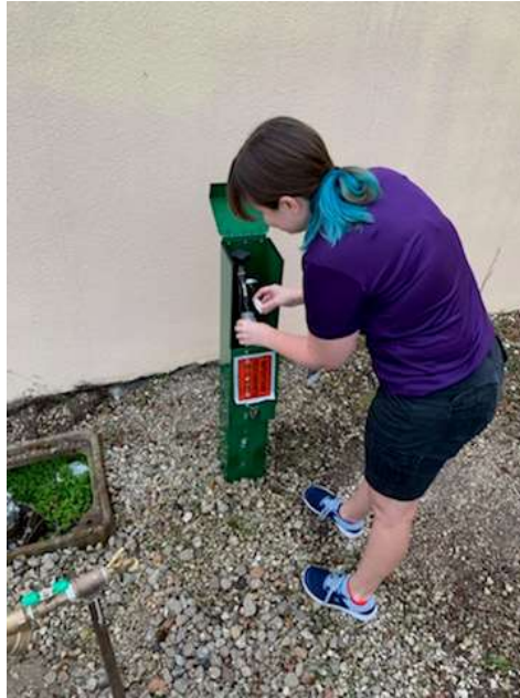
Photo of Lab Analyst Kerri Rodgers, Lab Tech, utilizing new sample station
