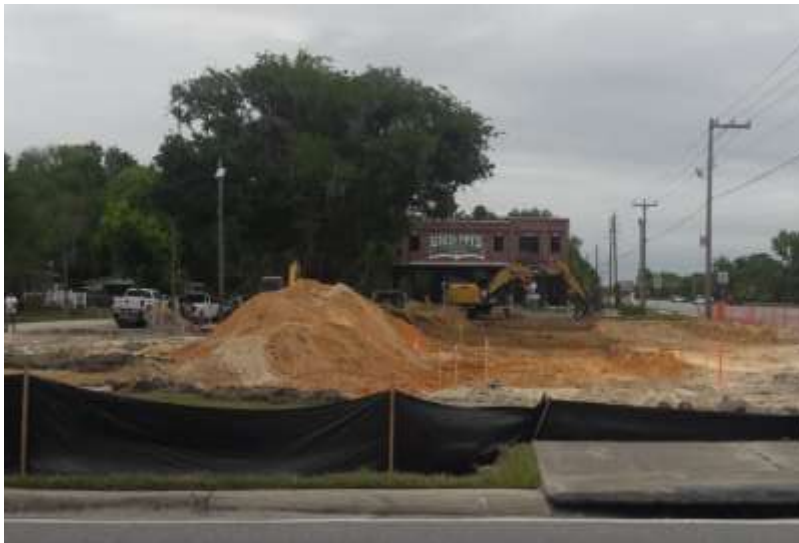
Photo of construction at the Giuseppe’s site.
