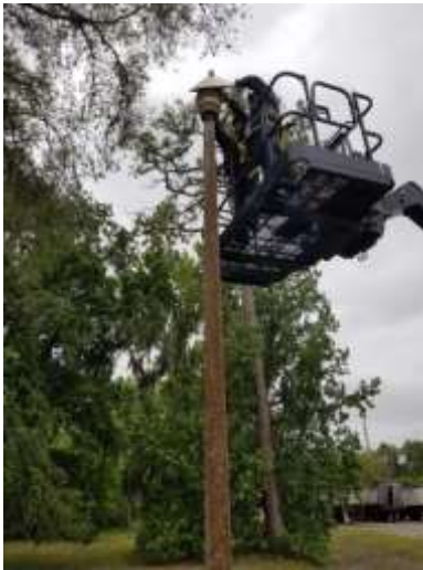
Photo of old light fixture being removed
