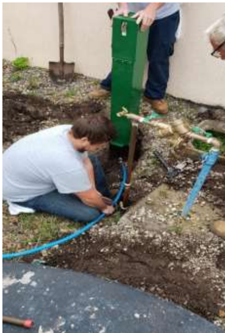
Photo of Crews installing a new water sample station
