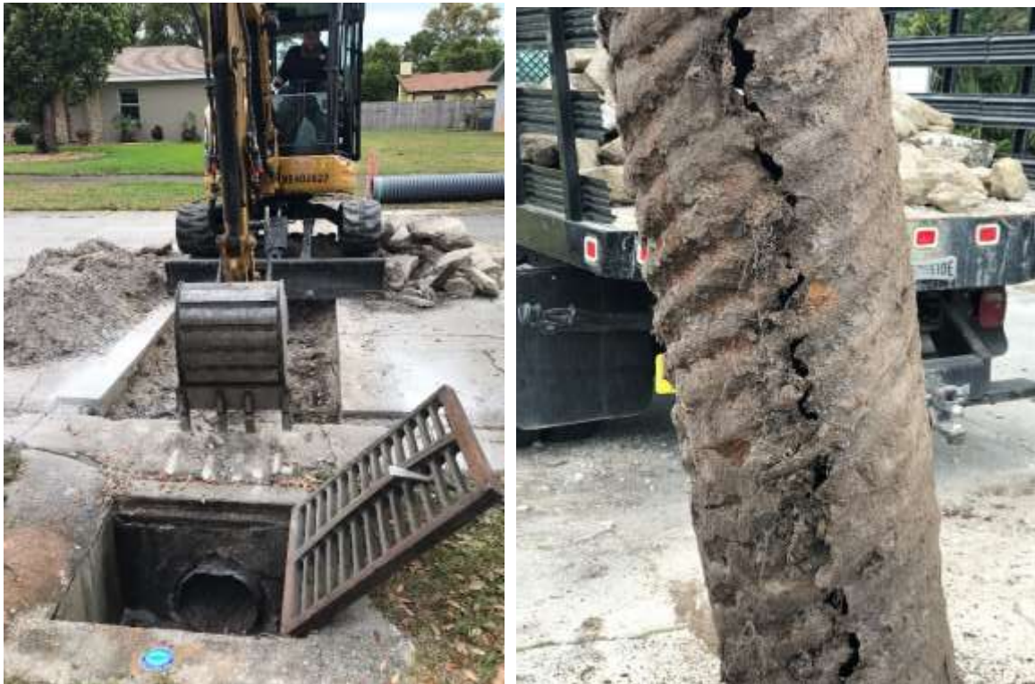
Photos of 5809 Wales Ave Metal Pipe Replacement Project
