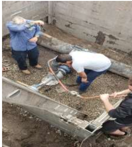
Photo of A New Potable Water Tap Installed on Williamson Blvd.
