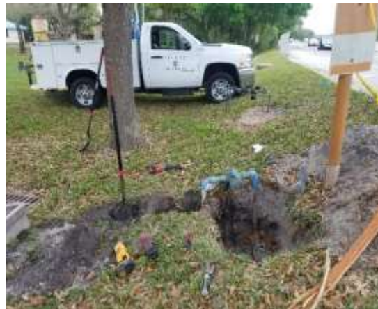
Photo of Williamson Lift Station Water Meter before Replacement
