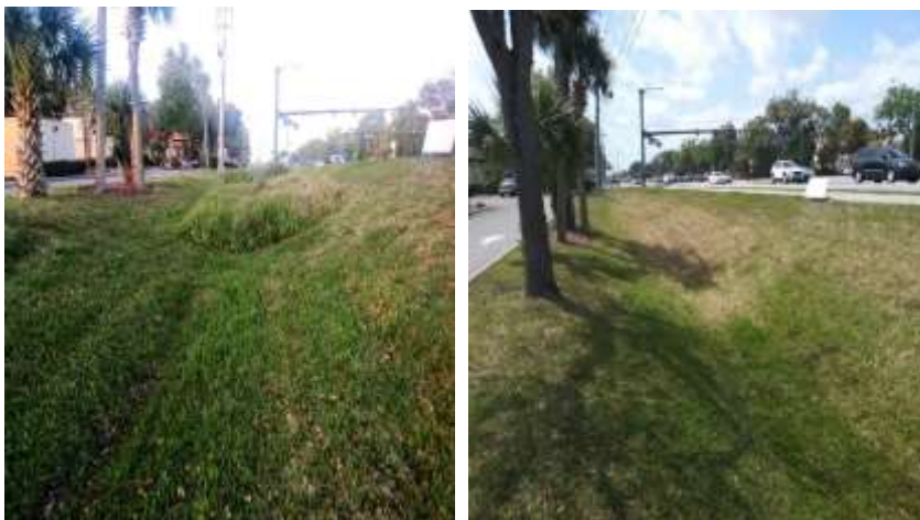
Photos of a Drainage Swale on Dunlawton Ave. Cleaned
