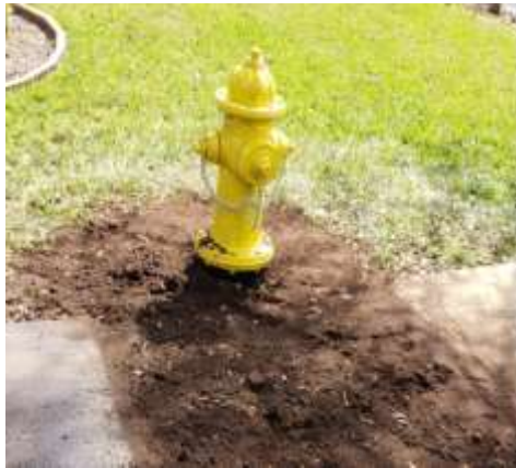
Photo of Fire Hydrant Replaced in Riverwood Subdivision
