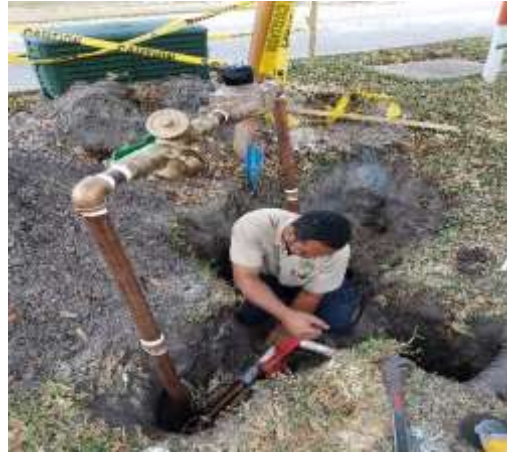
Photo of Crew Replacing Williamson Lift Station Water Meter
