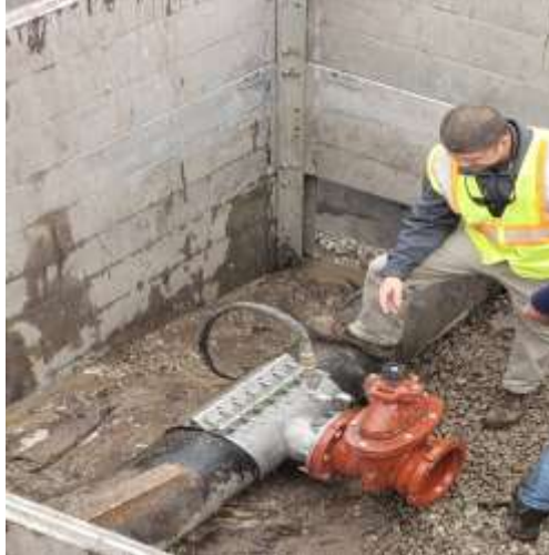
Photo of A New Potable Water Tap Installed on Williamson Blvd.
