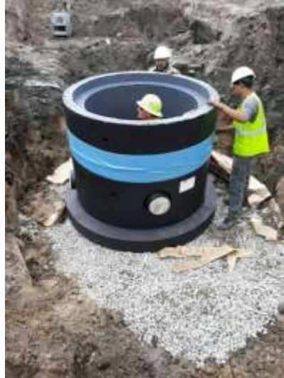
Developer Installing New Manhole Structures at the Springs Apartment Complex
