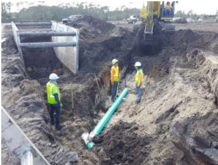
Developer Installing New Sewer Pipes at the Springs Apartment Complex
