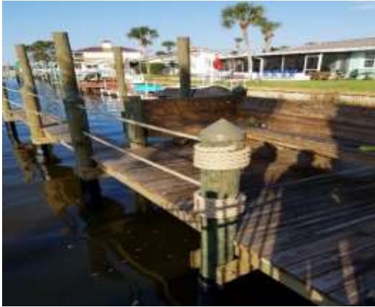
Photo of the dock before it was removed
