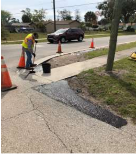
A photo of Hidden Lakes Dr. during repairs
