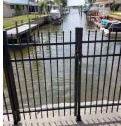
Photo of the dock after it was removed
