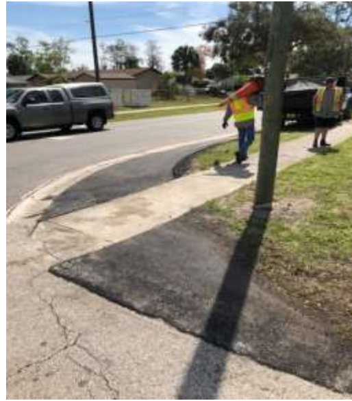
A photo of Hidden Lakes Dr. after repairs
