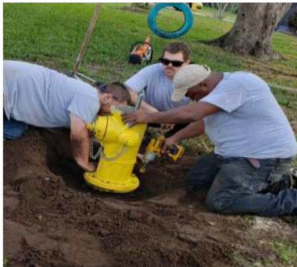
Crew Replacing Fire Hydrant on Viking Dr.
