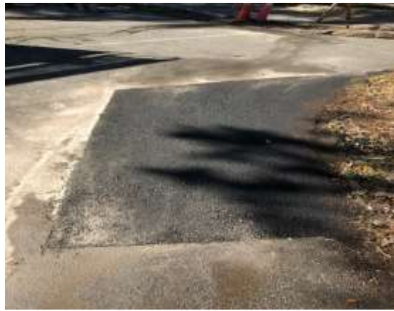
Annex Parking Lot After
